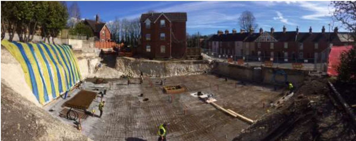
Workmen busy laying the foundations for the new Kimberly House
